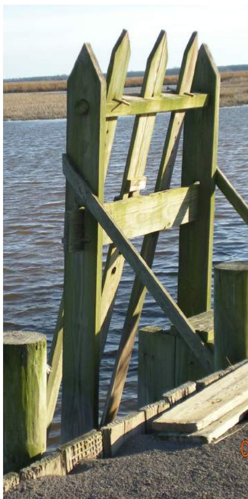
Combahee-Style Rice Field Trunk. Wooden structures, like this trunk, have a limited lifespan and are subject to repair and eventual replacement.
